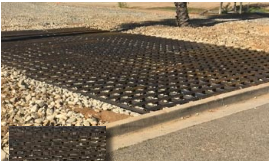
March Air Force Base Rumble strips 36' x 24' for military trucks exiting point to release mud from tires
